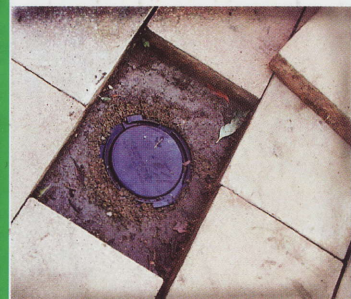
Installation under pavers
