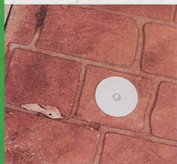
Installation through concrete.
